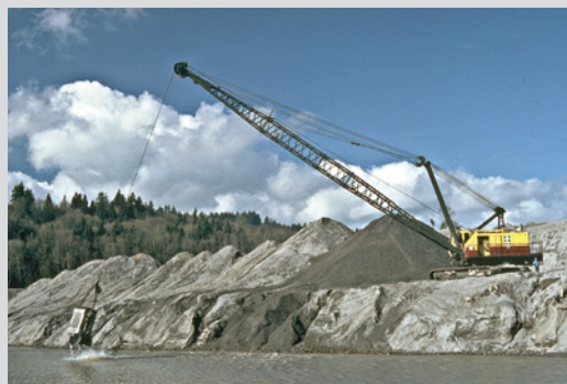
The U.S. Army Corps of Engineers dredged sediment from the Toutle (shown here), Cowlitz, and Columbia Rivers. By 1987, the volume of material removed was equivalent to a highway 12 lanes wide, 1 foot thick, stretching from New York to San Francisco. USGS photo by Lyn Topinka, February 5, 1981.
