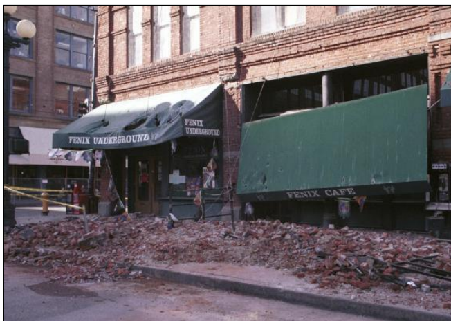
Figure 2. Historic buildings in Seattle's Pioneer Square damaged by the M6.8 Nisqually earthquake in 2001.
